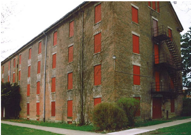
South Hall (BEFORE) – (North Hall similar), Antioch College, Yellow Springs
